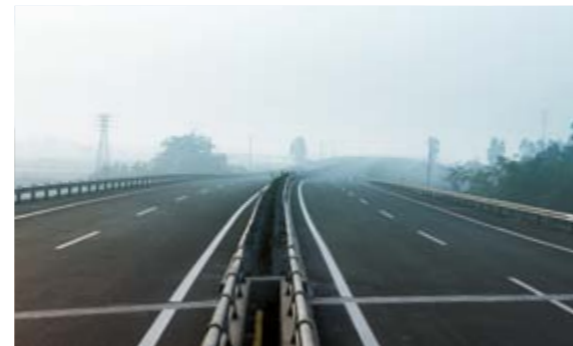
Noi Bai–Lao Cai Highway Construction, Vietnam
