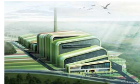
Construction of a Thermal Waste Incineration Plant, Krakow, Poland
