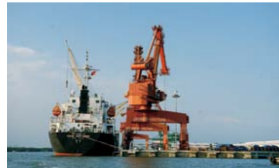
Exclusive Port for Vung Tau Cold Rolling Mill, Vietnam
