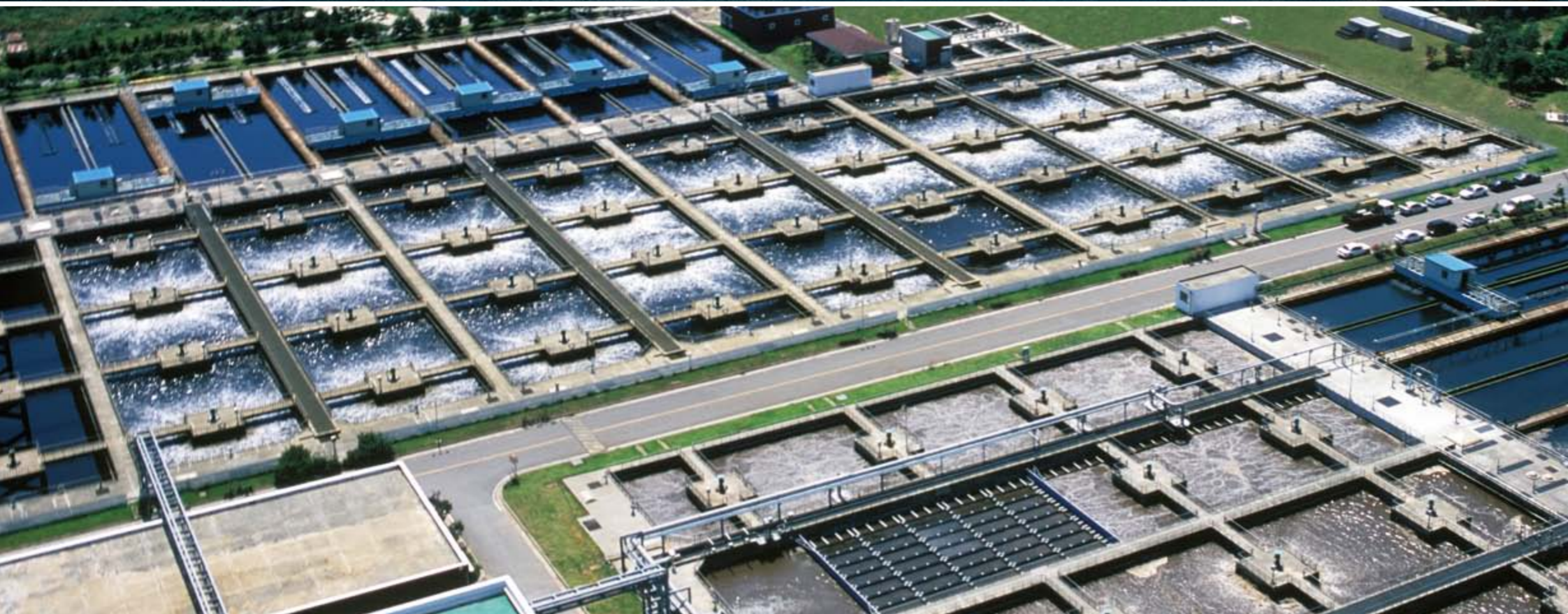
Gwangang Bridge, Busan, Korea (top) / Ansan Sewerage Treatment Plant, Korea (bottom)
