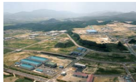
Chungju Company Town Infrastructure, Korea
