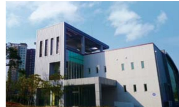
Cheongna Auto Clean Net Facility, Korea
