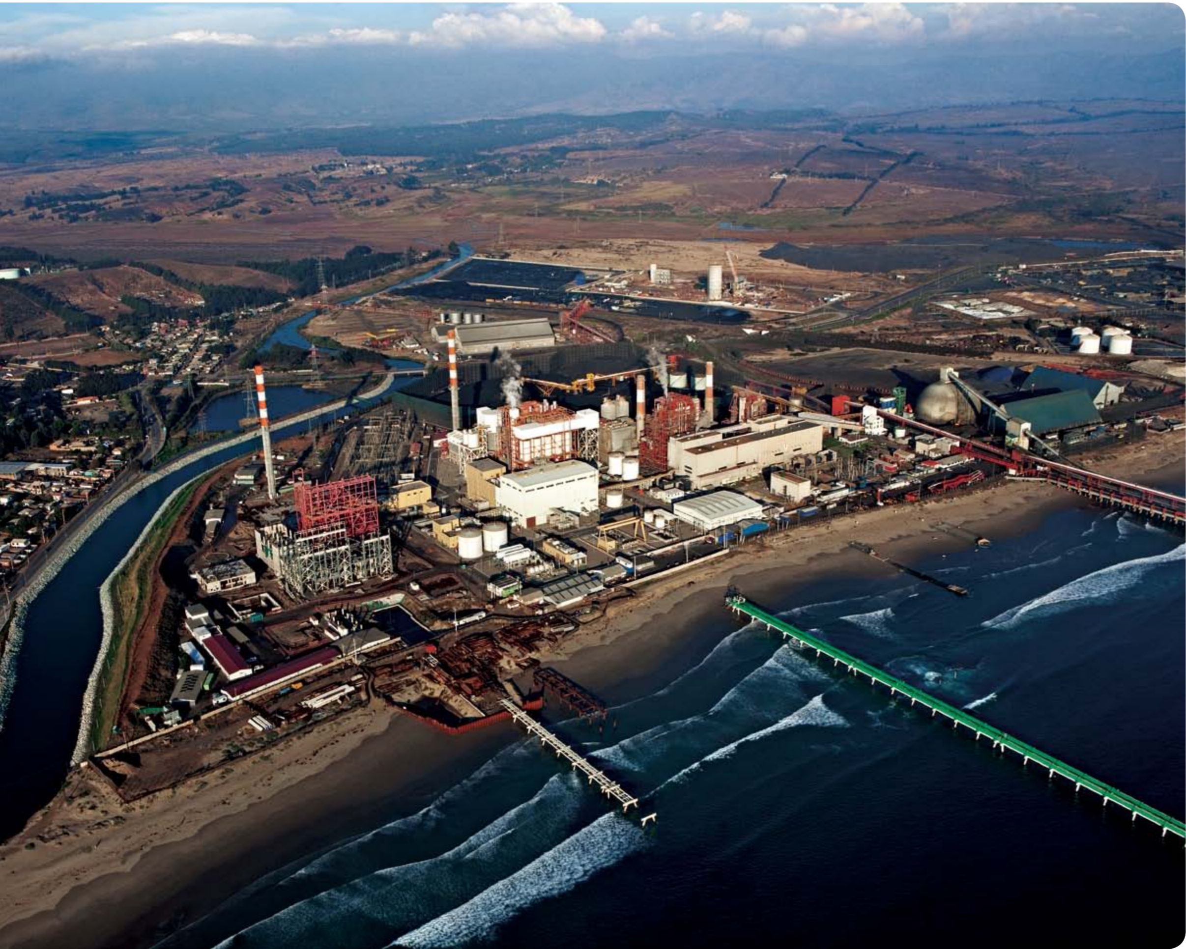
Nueva Ventanas Coal-fired Power Plant, Chile
