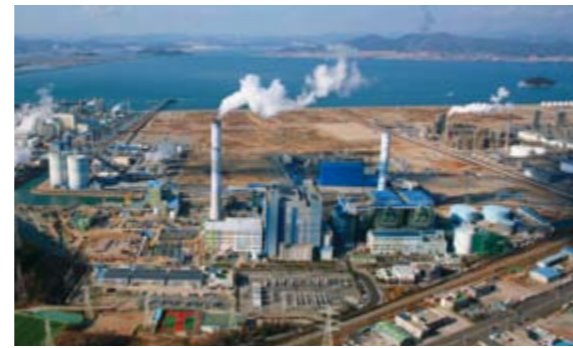
Yeosu Thermal Power Plant unit 1, Korea
