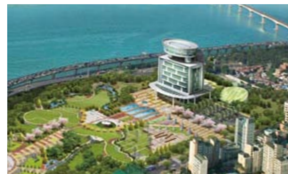
Seoul Combined Cycle Power Plant Units 1&2 civil engineering & construction, Korea
