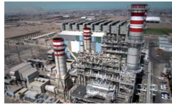
Chilca Uno Combined Cycle Coal-fired Power Plant, Peru
