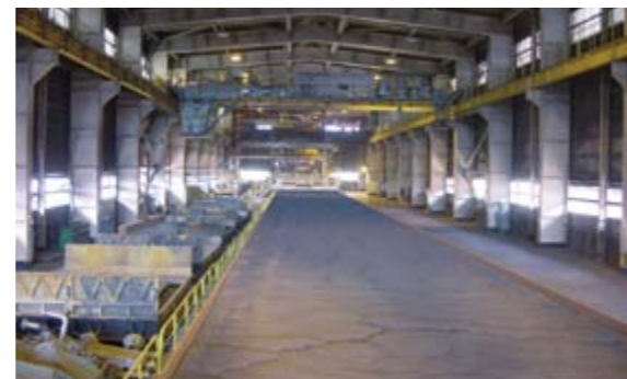
No. 3 Sintering Plant Revamping, Pohang Works, Korea
